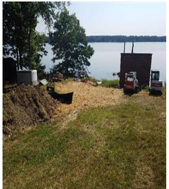
Fig 12: Erosion controls installed around cable house due to excavation. Viewing east. (7-26-19).
