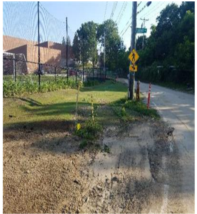
Fig 22: Vegetation growth along Colovos Rd. Viewing north. (7-29-19).
