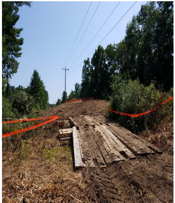
Fig 4: Stonewall WP-11 crossing. Viewing south. (7-25-19).
