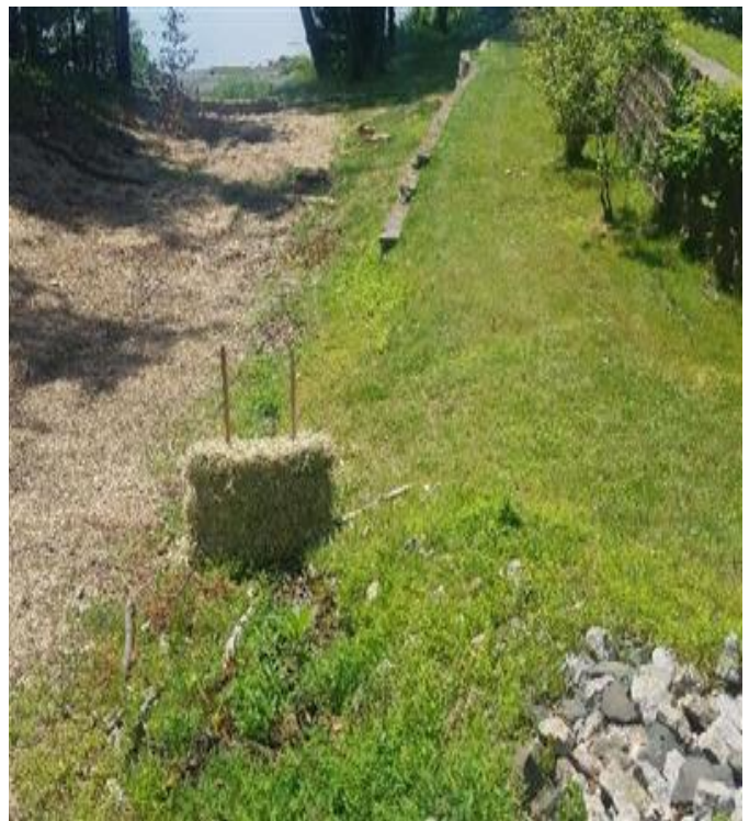
Fig 16: Additional erosion controls installed at Gundalow Landing. Viewing southwest. (7-26-19).
