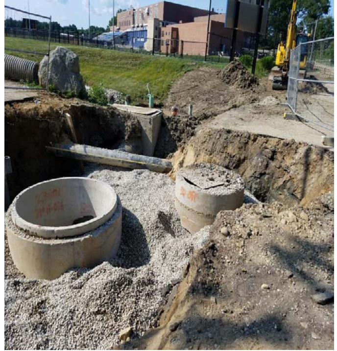
Fig 2: Placing manhole structures next to Colovos Rd. Viewing north. (7-25-19).
