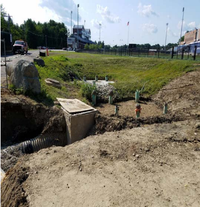
Fig 1: McCourt excavating through the rain garden. Viewing west. (7-25-19).
