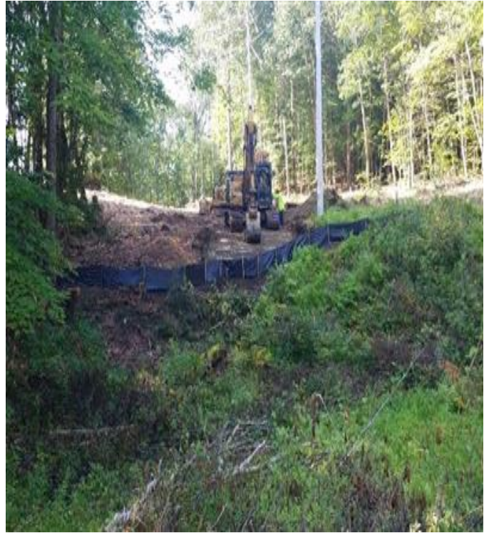
Fig 10: Building new access road to Str. 28. Viewing south. (7-26-19).
