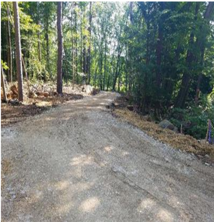
Fig 11: Access road to Str. 29, off of Mill road. Viewing north. (7-26-19).
