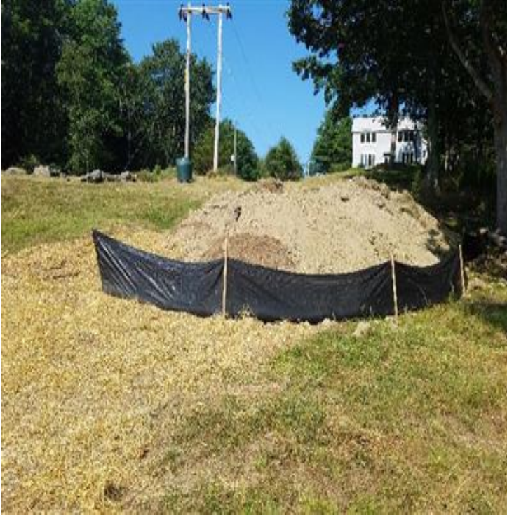
Fig 13: Stockpiled soil from cable house excavation. Viewing west. (7-26-19).
