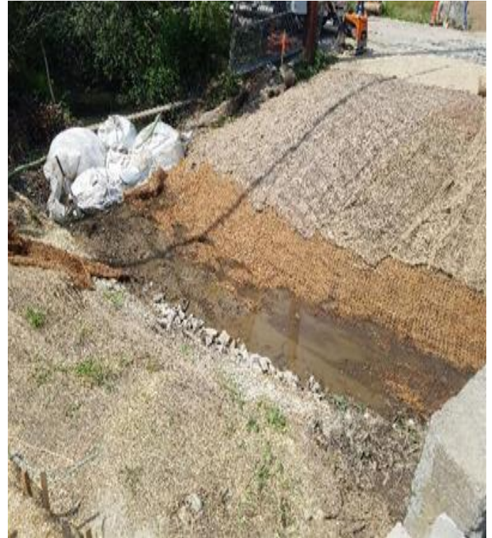
Fig 18: Installing coconut liner in College Brook. Viewing north. (7-29-19).
