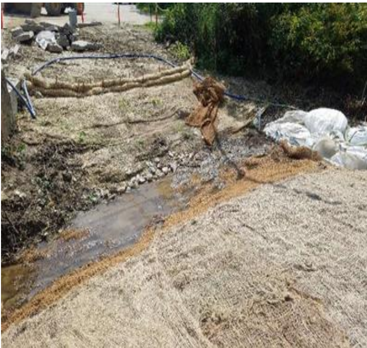
Fig 19: Installing coconut liner in College Brook. Viewing south. (7-29-19).
