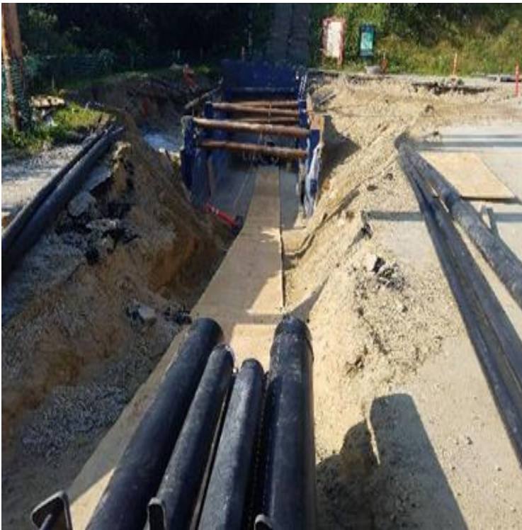
Fig 23: Prep work at jacking pit. Viewing south. (7-29-19).
