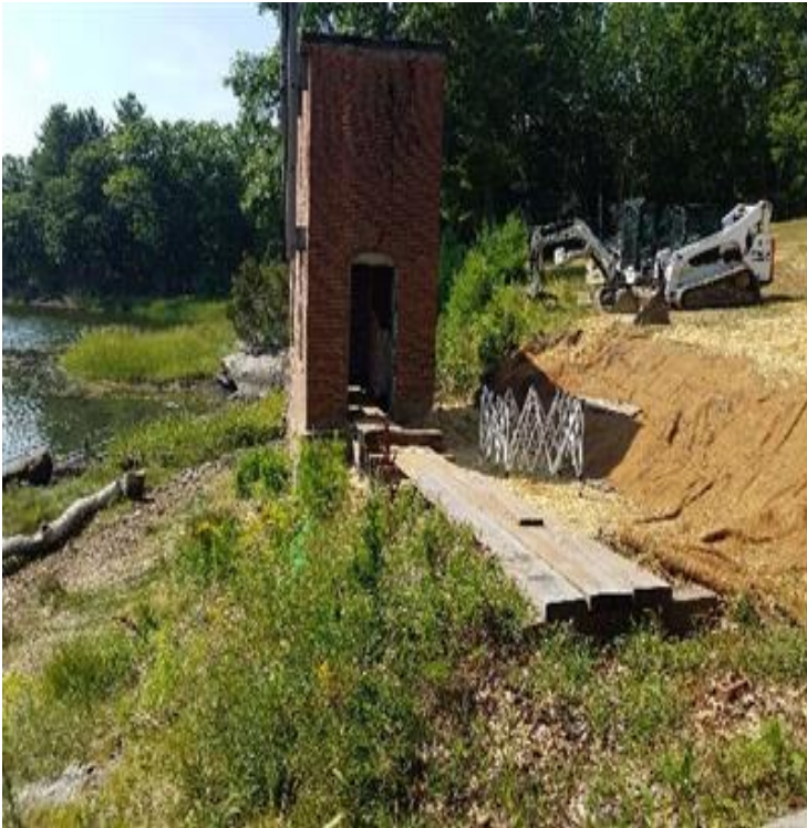
Fig 29: Cable house progress. Viewing south. (7-30-19).
