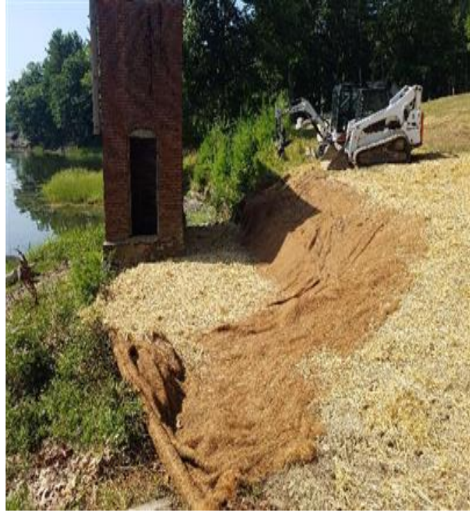
Fig 14: 4ft excavation around the cable house with erosion controls. Viewing north. (7-26-19).
