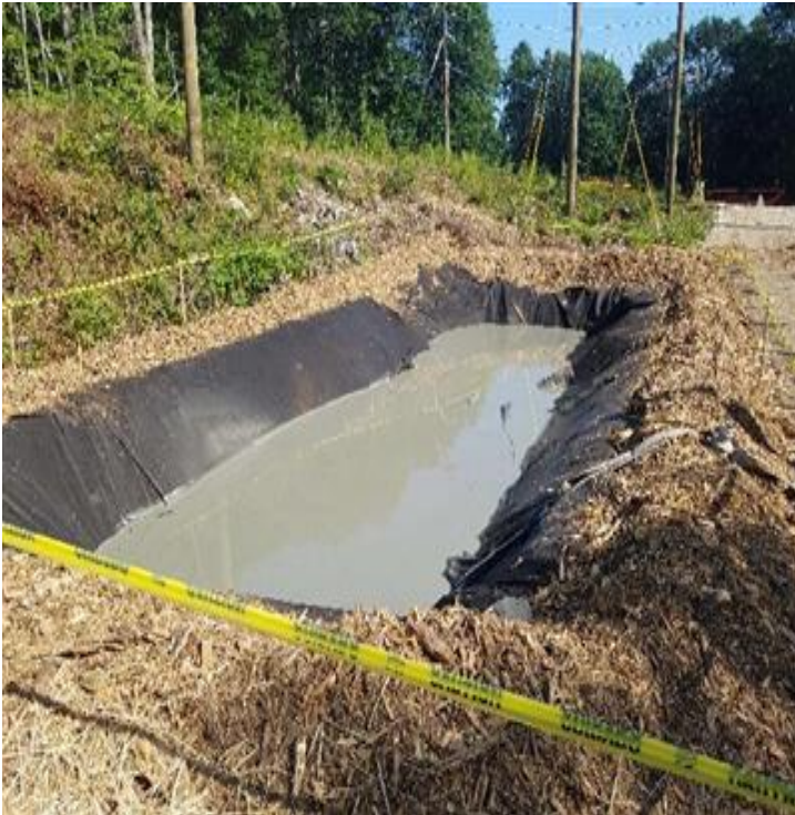
Fig 25: Dewatering basin next to Str. 32, lined with filter fabric. Viewing north. (7-29-19).
