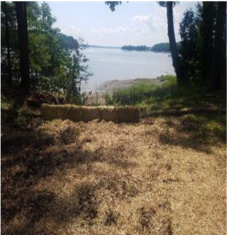
Fig 15: Additional erosion controls installed at Gundalow Landing. Viewing southwest. (7-26-19).
