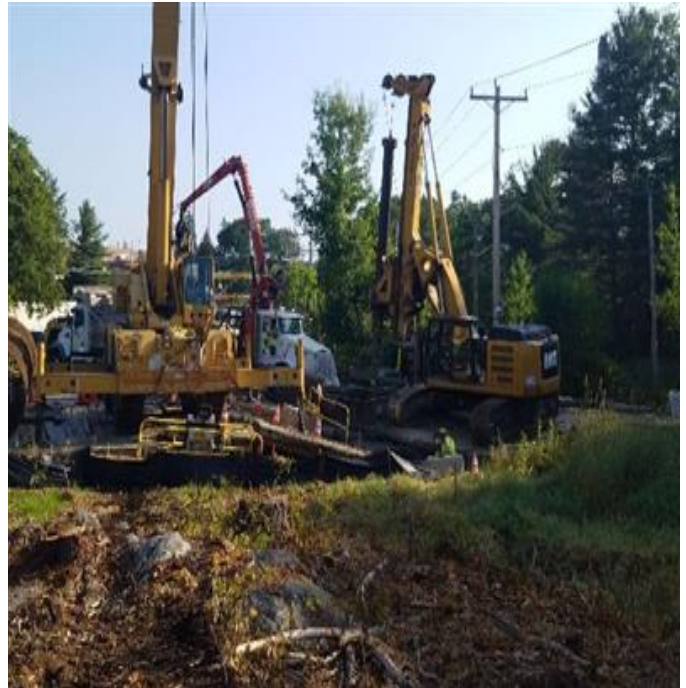
Fig 6: MJ drilling Str. 23. Viewing north. (7-26-19).
