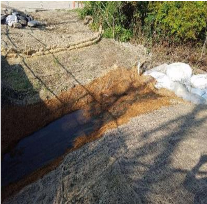
Fig 27: Continuing to install coconut liner in College Brook. Viewing south. (7-30-19).
