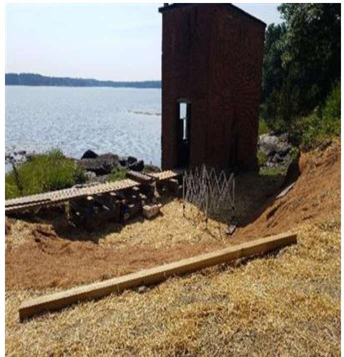
Fig 28: Cable house progress. Viewing south. (7-30-19).
