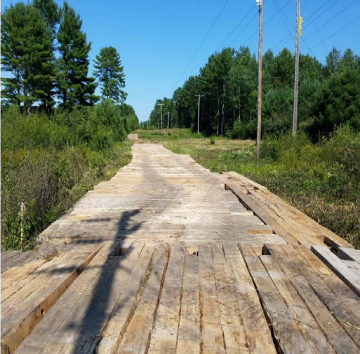
Fig 5: Timber matted access route through wetland DW56 towards Str. 49. Viewing east. (7-25-19).
