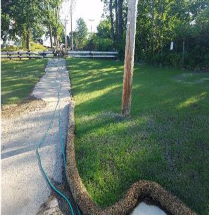
Fig 21: Vegetation growth south of steam pipe. Viewing north. (7-29-19).
